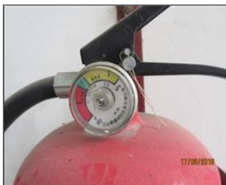
External photo(s) of the production unit(s) Fire extinguishers in good condition.JPG
