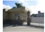
factory entrance gate and the security guard room.JPG
